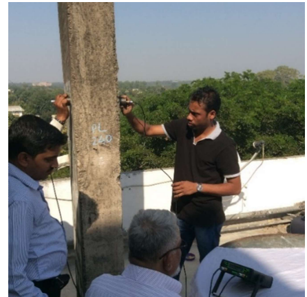
CONCRETE COLUMN TESTING
