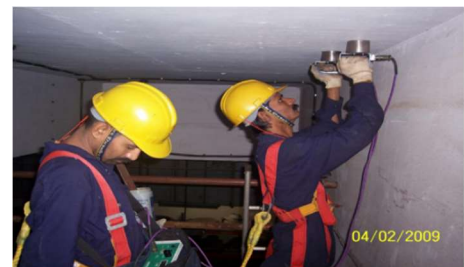
SURFACE PROBING OF ROOF SLAB
